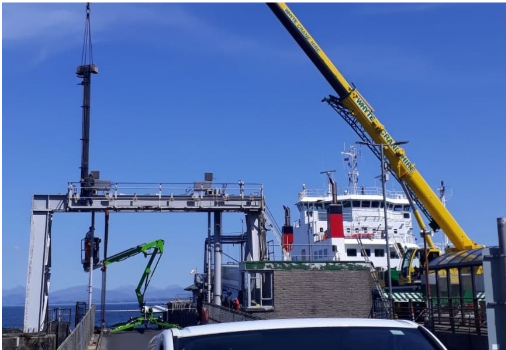
Replacing hydraulic cylinder - Craignure
